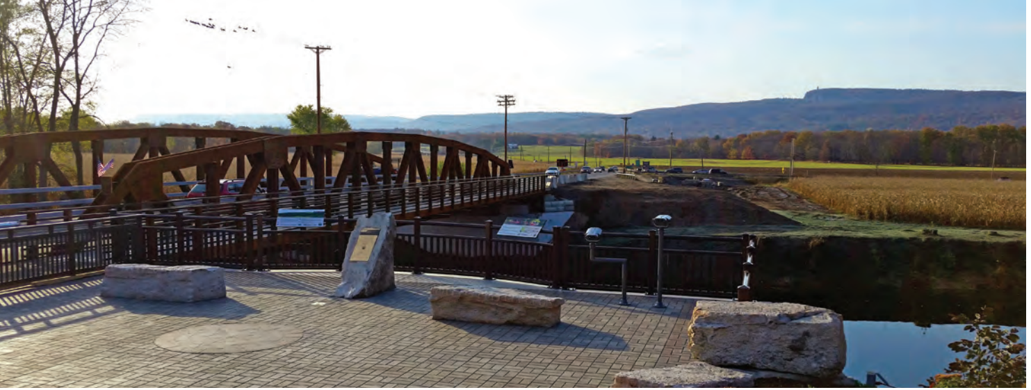
Carmine Liberta Bridge Viewing Platform, New Paltz
